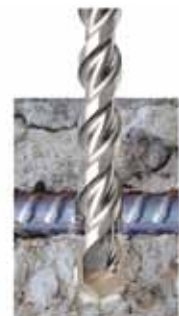
Rebar Step 3 Hammer Drill
